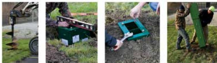
and contractors alike. **It's constructed with 14 gauge steel and only available for 12" pedestals.**
