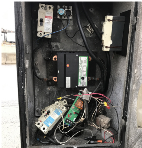
An outdated lighting control cabinet along the Skyway Bridge in Chicago, Ill.
