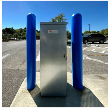
Gladstone, MO This Milbank pedestal supplies power for the Chase Bank ATM parking lot kiosk.
