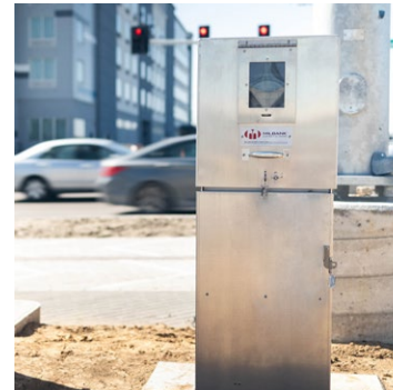
St. Louis, MO Power distribution and controls cabinet provides power for traffic lights throughout the city of St. Louis. The unit shown was designed to meet specific guidelines set by MoDOT, and serve as the standard unit for traffic controller cabinets.
