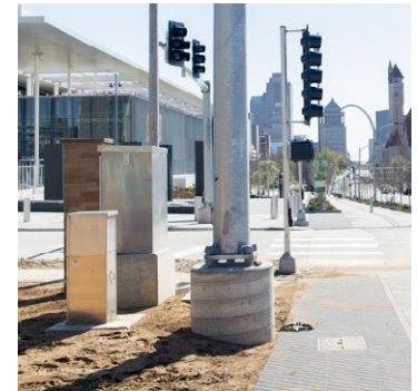
St. Louis, MO Power distribution and controls cabinet provides power for traffic lights throughout the city of St. Louis. The unit shown was designed to meet specific guidelines set by MoDOT, and serve as the standard unit for traffic controller cabinets.
