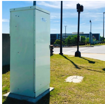
Atlanta, GA Intersection near the Atlanta Braves stadium in Atlanta, GA uses 16-inch exposed meter pedestal to manage the intersection traffic control.
