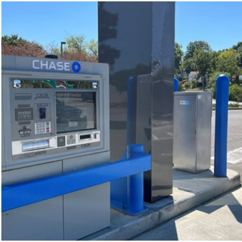
Gladstone, MO This Milbank pedestal supplies power for the Chase Bank ATM parking lot kiosk.
