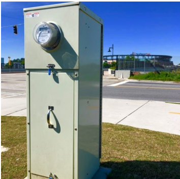
Atlanta, GA Intersection near the Atlanta Braves stadium in Atlanta, GA uses 16-inch exposed meter pedestal to manage the intersection traffic control.
