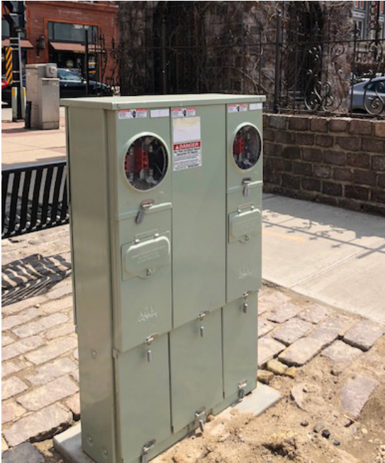
K6342 installation distributes power to cellular repeater.
