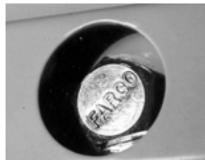
Penta Bolt locking mechanism
